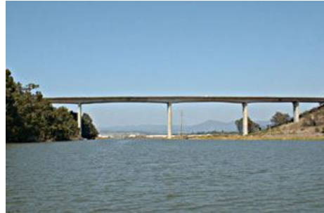
Butler Bridge Fixed
