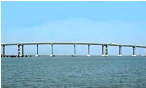
Highway 37 Fixed Bridge
