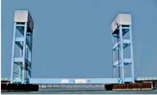
Mare Island Bridge
