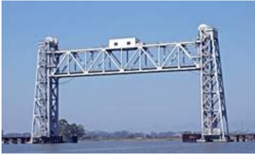
Brazzo Train Bridge
